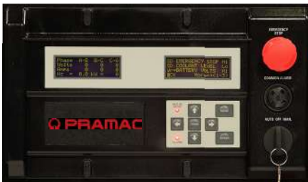
Digital H Control Panel—Dual 4x20 Display
